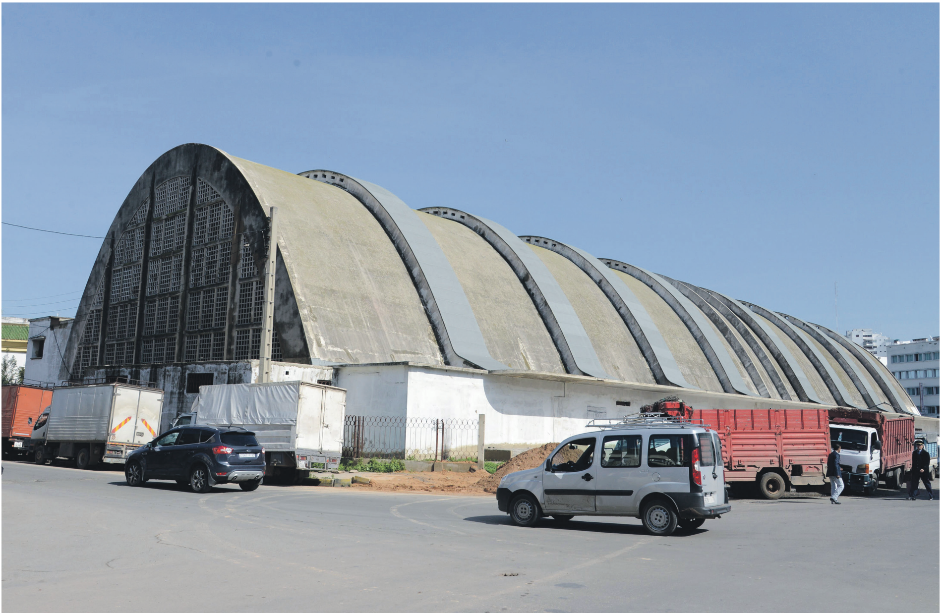
The re-establishment of the former wholesale market building in order to convert it into a socio-sports area will require a budget of 50 million Dirhams (Ph. L'Economiste)
