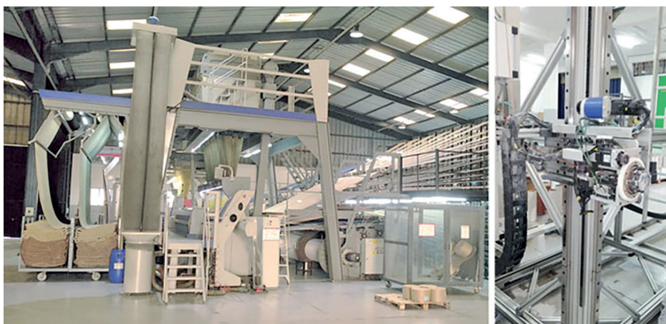
An Alpha 500 weaving machine of German origin. It is installed in one of the three workshops of the Aleptex company. This carpet manufacturer is headquartered in the Lissasfa industrial zone in Casablanca and is one of the plaintiffs against "massive imports" from China, Egypt, and Jordan (Ph. F.F.)
