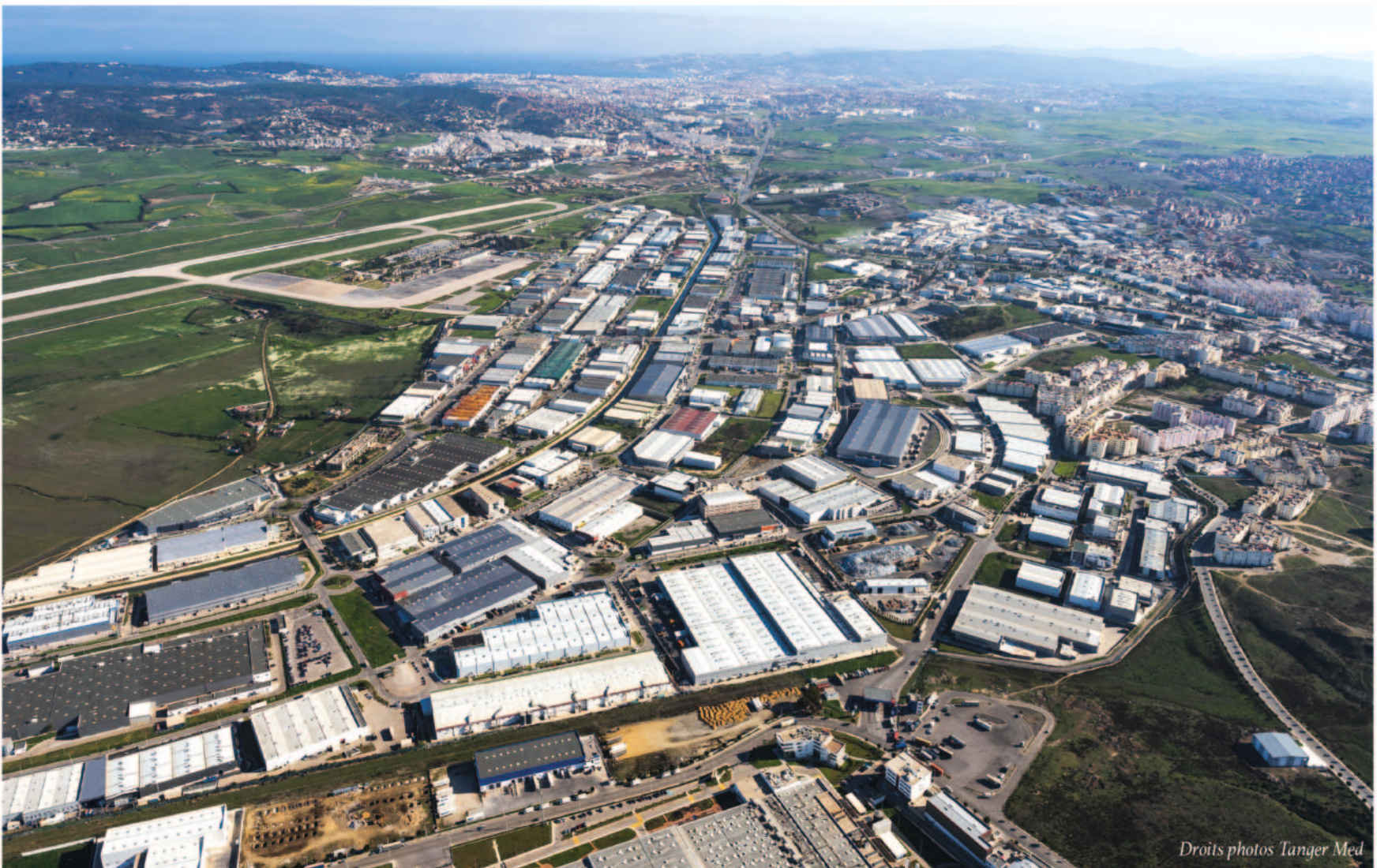
Plateforme industrielle Tanger Med.
